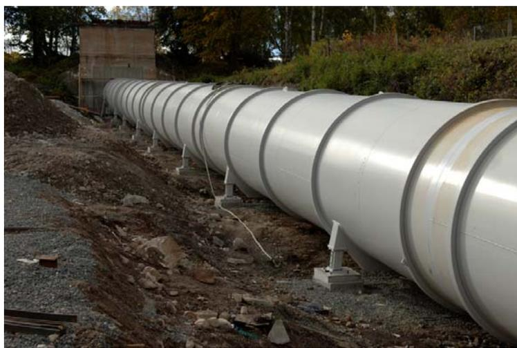
Figure 4. Straight penstock down-stream surge chamber
