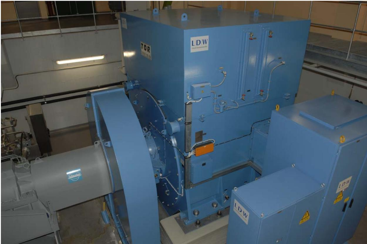
Figure 7 The synchronous generator. The cooling air is circulated through heat exchangers at top of which one is supplying warm water to a large accumulator tank. That water is used to heat the building mainly during standstill at nights and weekends.
